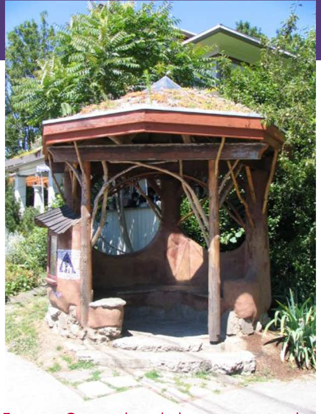
Eugene, Oregon bus shelter, no poster ads, open design, "live" roof, made with local cobb material. (Photo: Michelle Saville)
